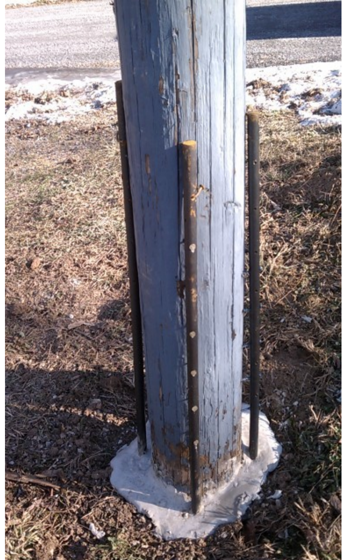
Repaired Swing-gate latch post
